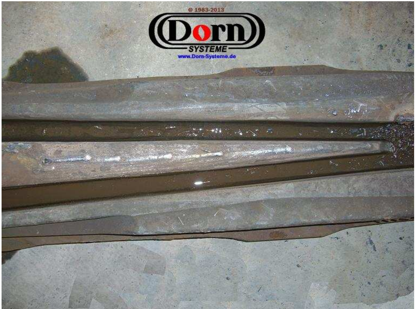
Two area welding at frog part, for best edges
